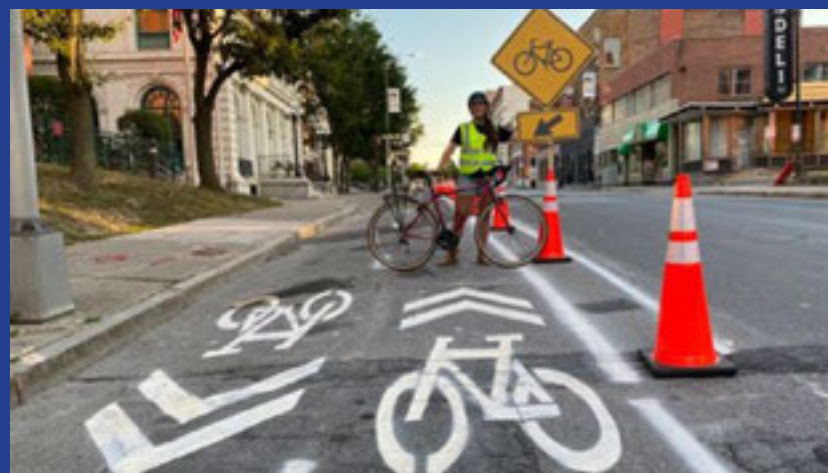
Image 58. Temporary Curb Extension Installation
