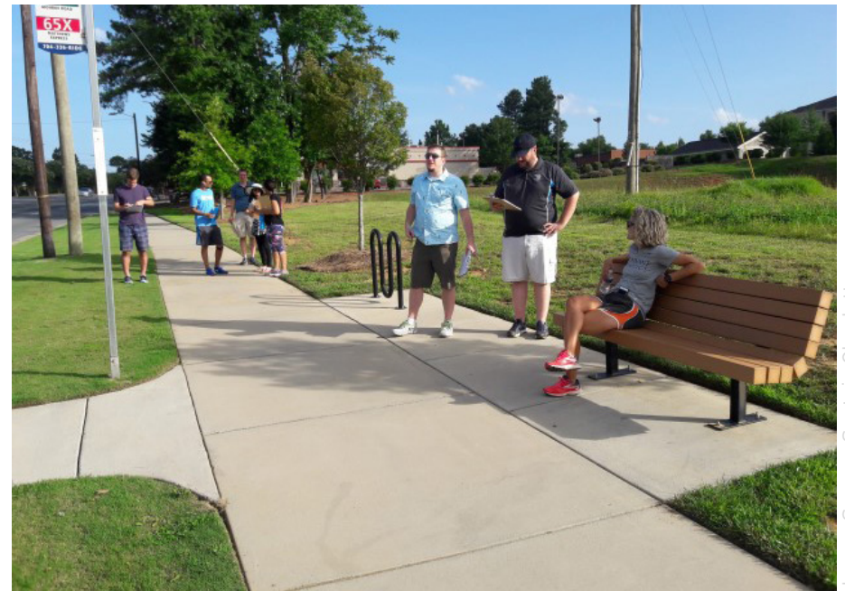
An accessible, comfortable bus stop with an ADA pad, sidewalk connection, bench, and bike rack, supporting safe and convenient transit access.
