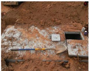
The septic tank is a two piece concrete box, sealed at the joints to prevent water seepage. It is placed just below ground level on an undisturbed bed of soil and leveled carefully. The home's wastewater supply line is connected to it. There are two access lids on the top which allow access for inspection and pumping of effluent.
