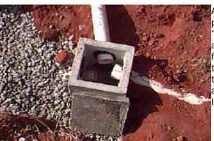
After leaving the septic tank, the effluent is piped to a distribution device, in this case a "dropbox", which is carefully leveled. There are two pipes leaving this box, one to the first trench, the second, which is higher, to the second trench. This allows the first trench to fill before the second. Another box allows the second trench to feed before the last.
